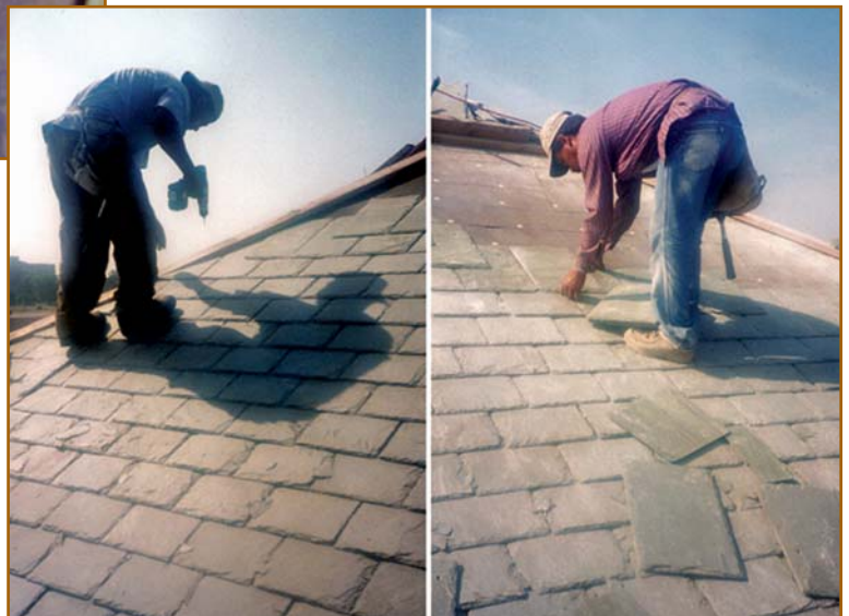
Figure 18 – It is a mistake to walk on a slate roof during installation.
